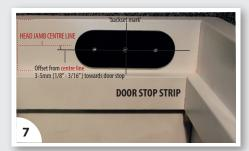
7. Open the door, then continue the 'backset mark' onto the underside face of the head jamb, towards the door stop strip.
